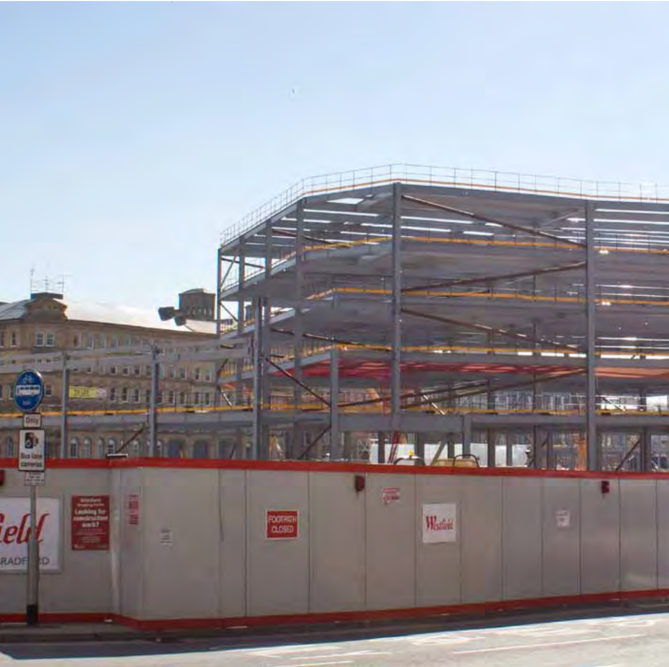
Westfield Broadway on site (2014)
