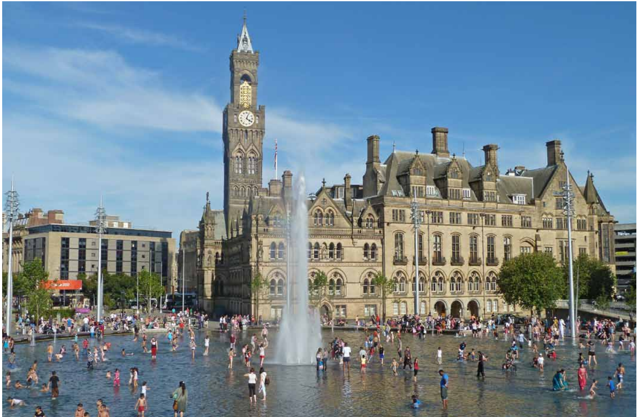
Bradford City Hall and City Park
