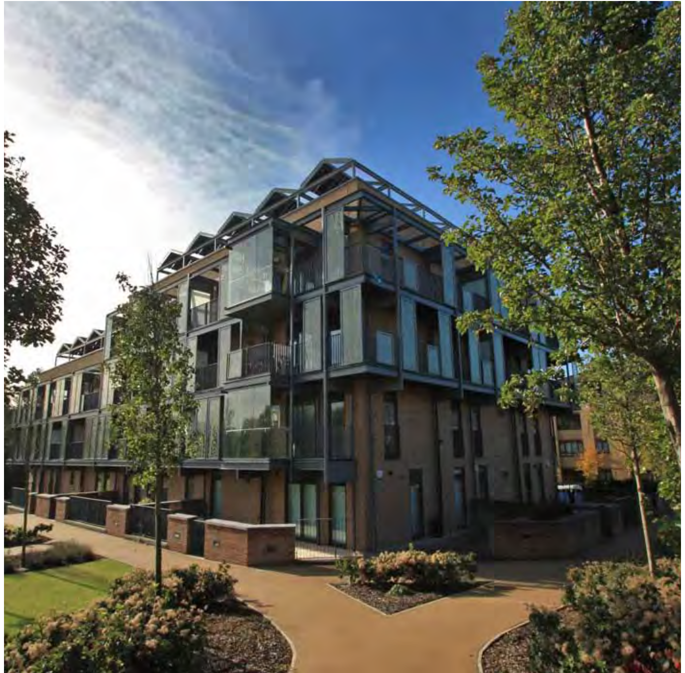
New city living to high design standards. Vizion development, Milton Keynes
