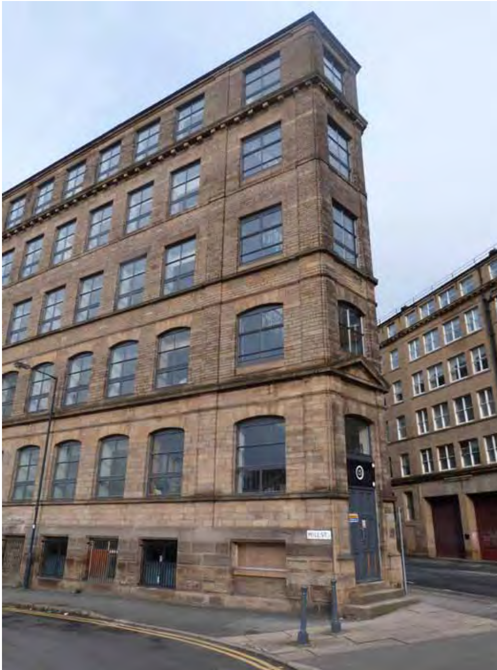
102 Recent residential conversion at 15-17 Canal Road Bradford
